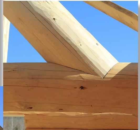
Mitered joinery at the bottom of the rafter. Looks great, and the angles are exactly what the engineers want to resist thrust.
